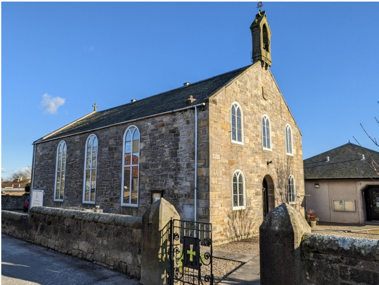
The former Strathkinness Parish Church, 2023. (B. Rhodes)
