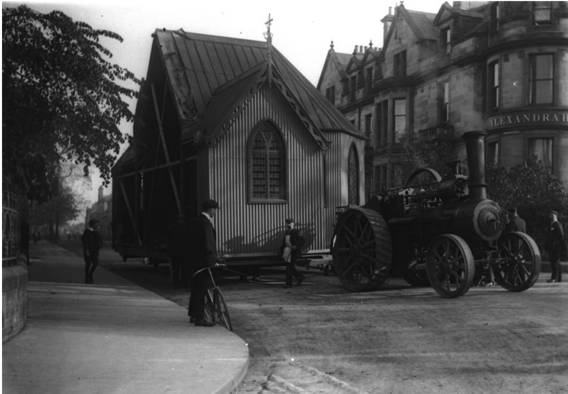
The original iron Church of St James being removed in 1909. (Source: University of St Andrews Library, GMC-F-95. Available at: https://collections.st-andrews.ac.uk/item/st-jamess-church-st-andrews/8269 )
