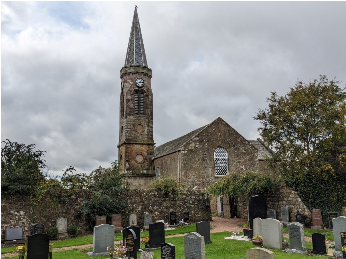
Kingsbarns Parish Church, 2023. (B. Rhodes)
