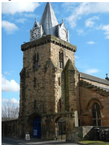
Fig 5. Parish Church of St Peter, West Tower
