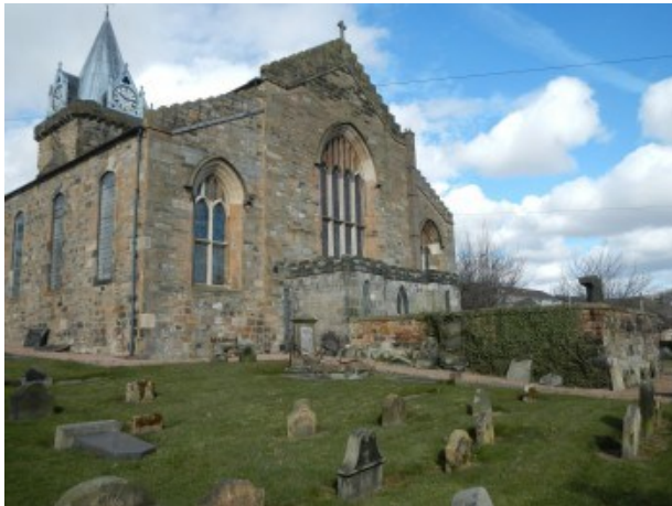
Fig 13. Inverkeithing Parish Church from the South East (R Fawcett, 2012)
