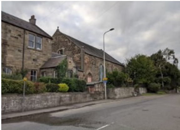
Fig 11. St John's, Inverkeithing (Bess Rhodes)
