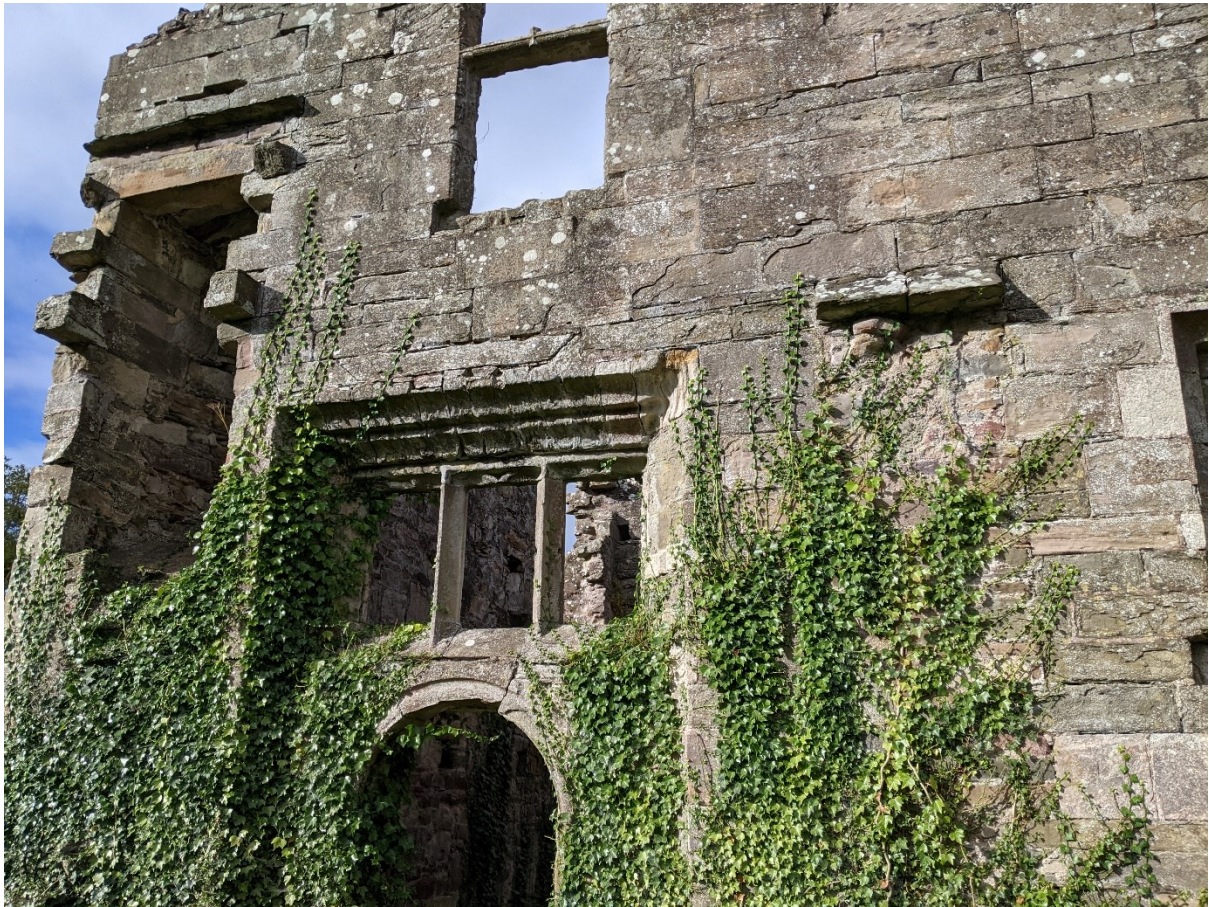
The former abbot’s house, with post-Reformation alterations into a laird’s house. (B. Rhodes)
