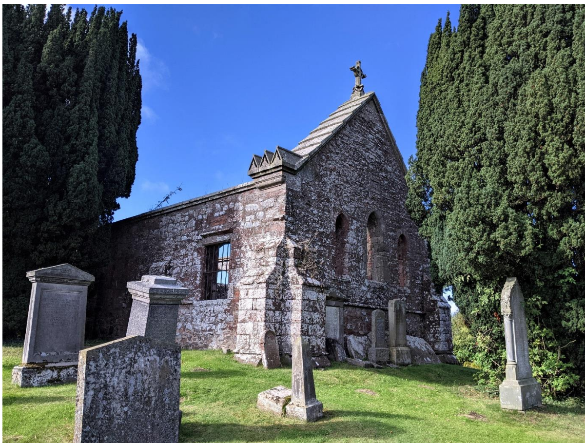
Exterior of east end of Abdie Old Parish Church. The buttress on the corner is medieval. The decoration on the gable is nineteenth century. (B. Rhodes)
