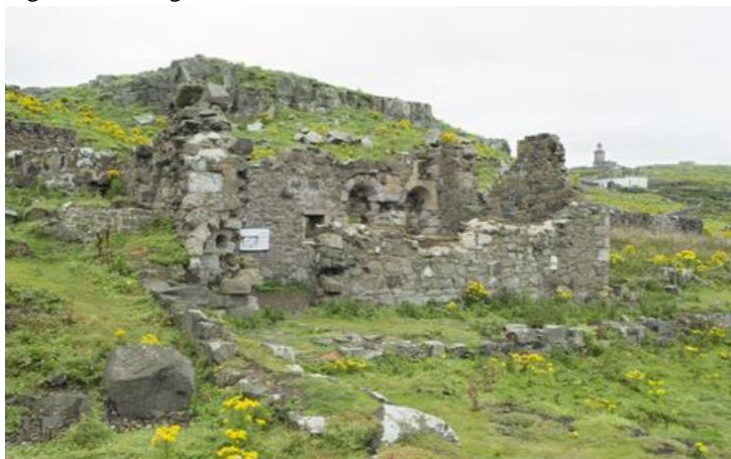
Fig 3. West range, view from southeast © Historic Environment Scotland. 19
