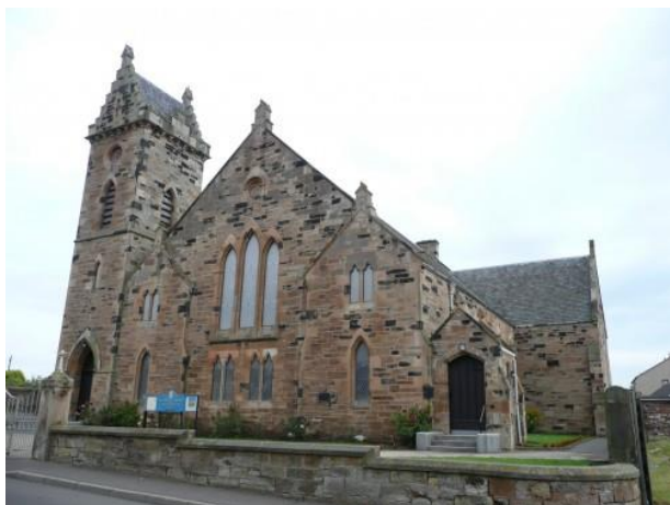
Fig 17. Cellardyke Parish Church, © Copyright 2021, SCHR Ltd. 117
