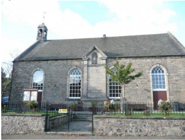
Fig 8. Aberdour Former Parish Church (@ Ewan Malecki (October 2007)). 62
